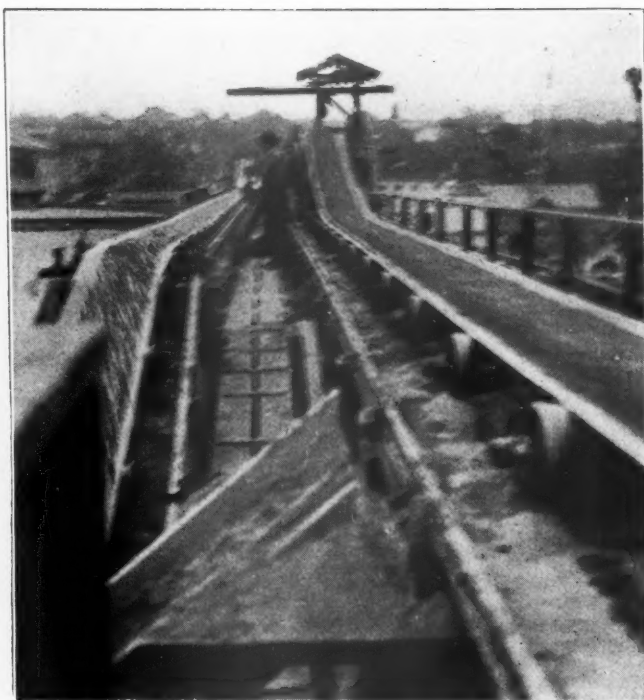
Conveyor Feeding Bins
